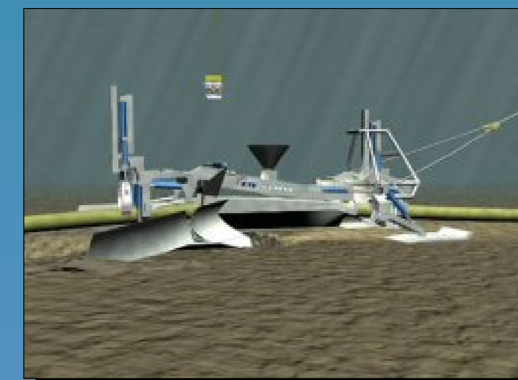
Plow being pulled along pipeline, creating trench for pipeline
